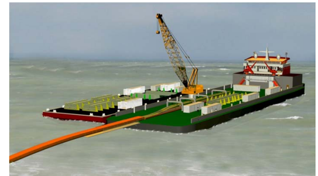
Offshore Pipe Assembly
