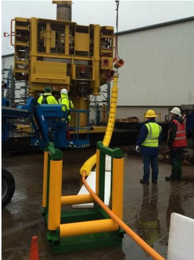
Wellhead/Tree Interface
